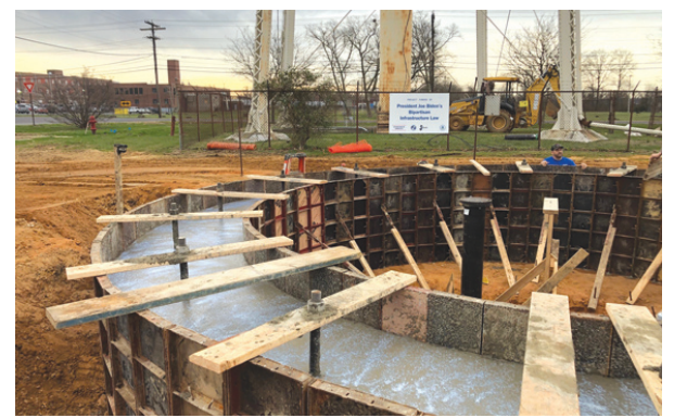
(above) Ringwall – Outer ringwall foundation encompasses the pilings for the tower.
