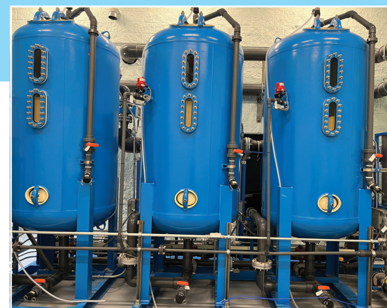
The Nitrate Removal Treatment system at the Love Lane Water Facility began operation in December 2022.
