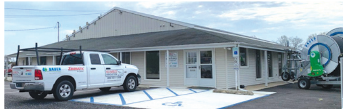
Sussex Irrigation opened their business at the corner of Highway 77 and Polk Lane.
