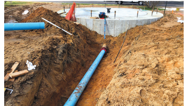
(below) Water line to provide water to the tower is installed.
