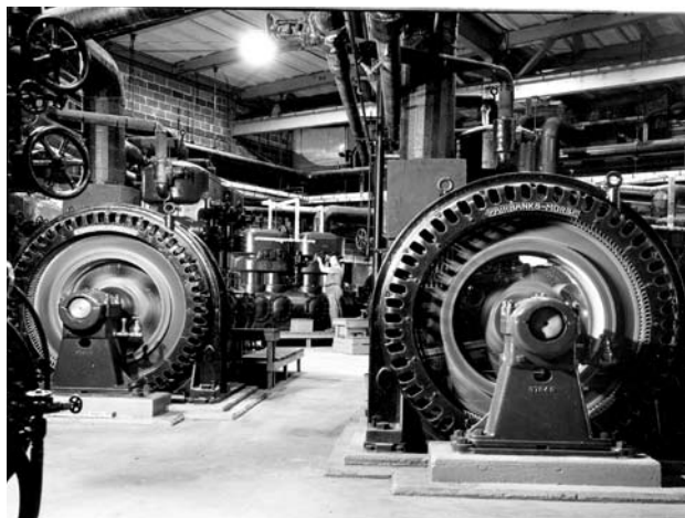
Refrigeration compressors
