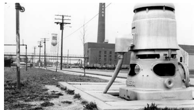
Deepwell pump that supplied water to either the Seabrook Farms plant itself or Seabrook Village. The Seabrook Farms water tower in the background
