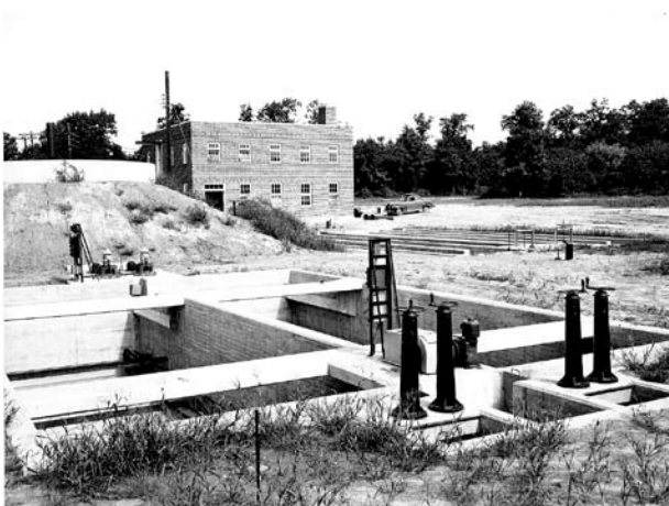
Seabrook Wastewater Treatment Facility
